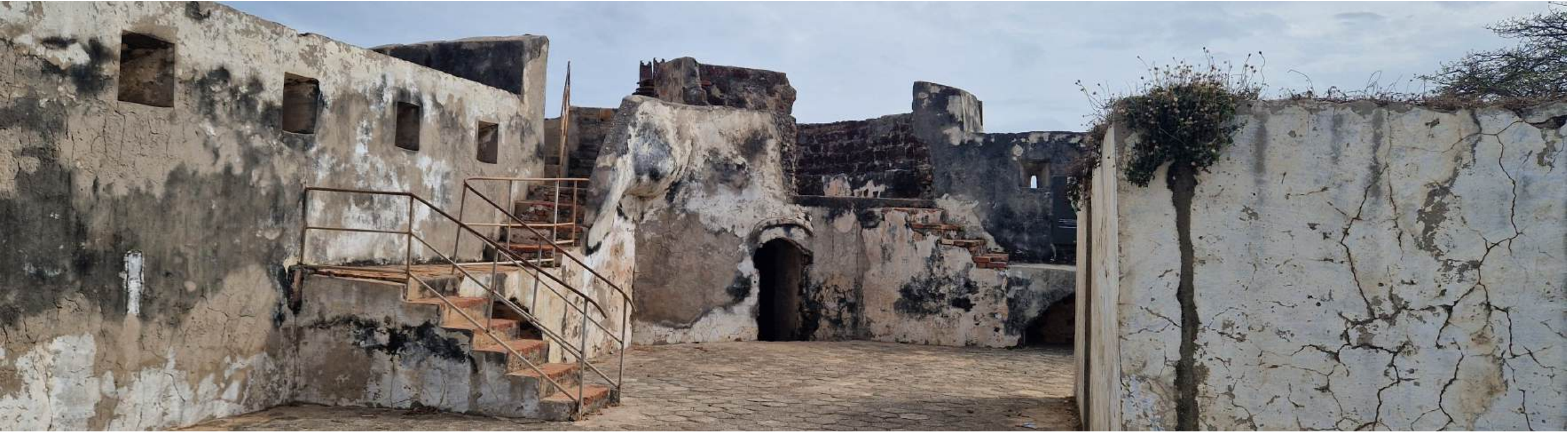
Figure 12 : Fort Bullen interior, showing the need for significant consolidation, safety and conservation measures (Photo dated 18 th June 2024)
