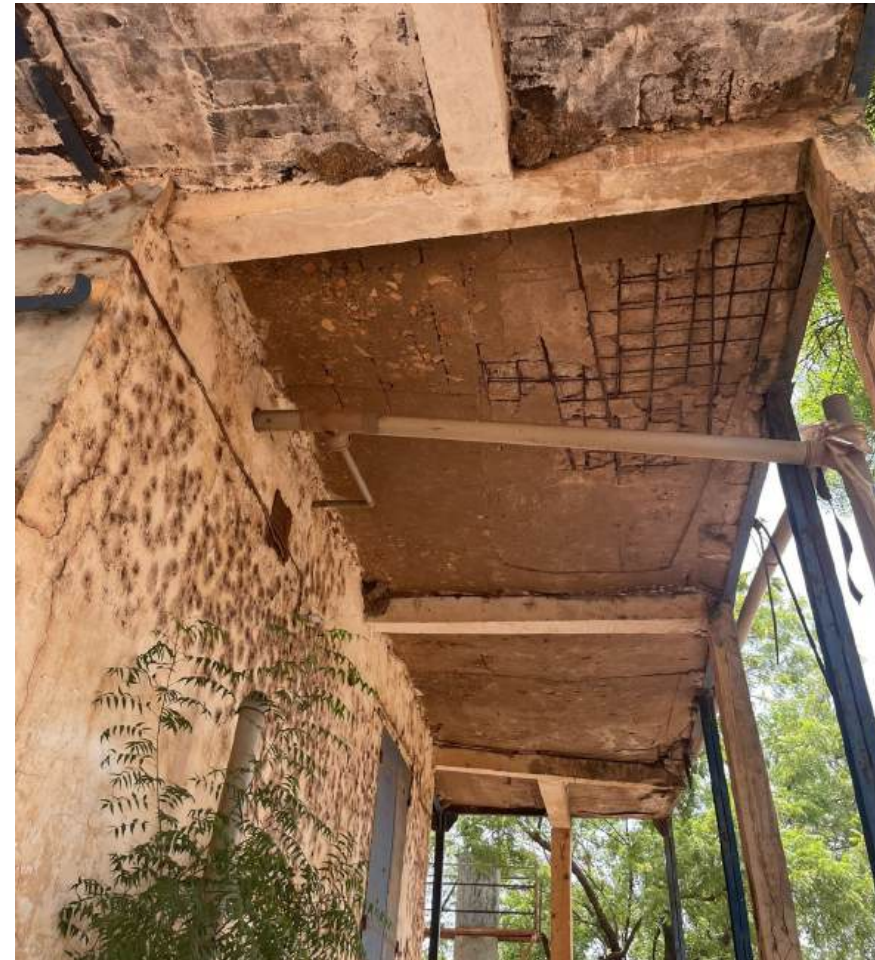
Fig. 13 : Traditional Building - Deteriorated ceiling to be rehabilitated
