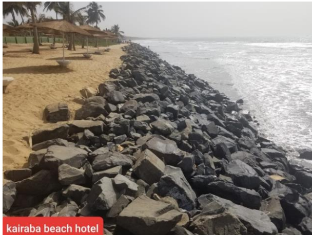
Picture 1 : Beach protection riprap at Kairaba Beach Hotel
